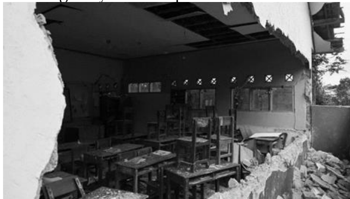
Figure 2. School in Cianjur, West Java, That Collapsed after Being Shaken by Earthquake
