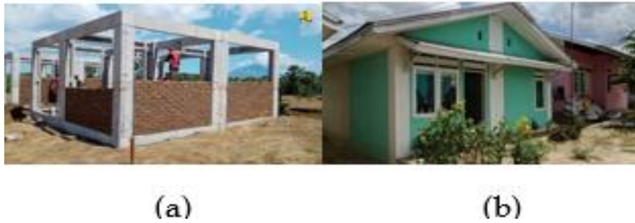
Figure 4. An Example of House Construction Using Methods of Risha, From Early Construction (A) to Its Final Result (B)
