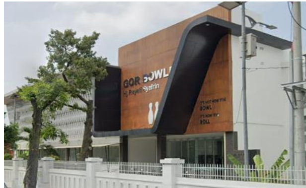
Figure 10. Front View or Entrance of Bowling Sports Hall (Source: Syahputra, 2025)
