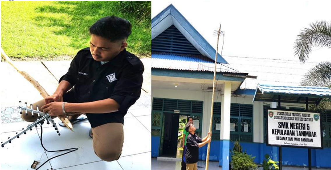
Figure 4. Antenna Installation Process
